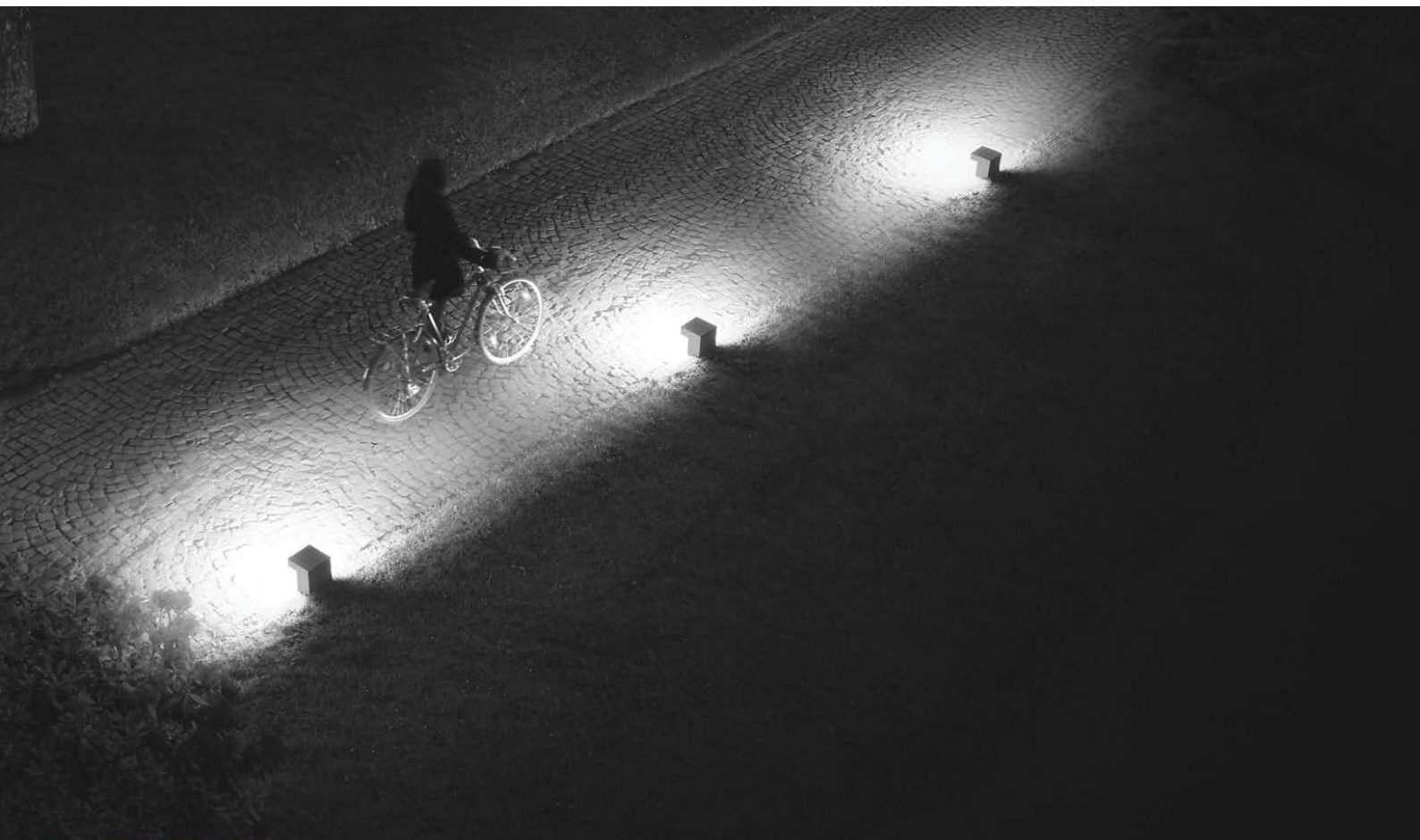
LED on-ground luminaires with flat beam light distribution for illuminating ground surfaces
